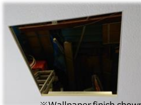
⑦ Paint or apply wallpaper
