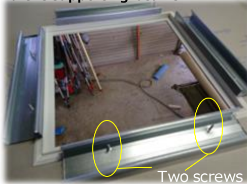
Sandwich the frame between the ceiling and the supporting beams
