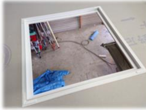
Sandwich the frame between the ceiling and the supporting beams
