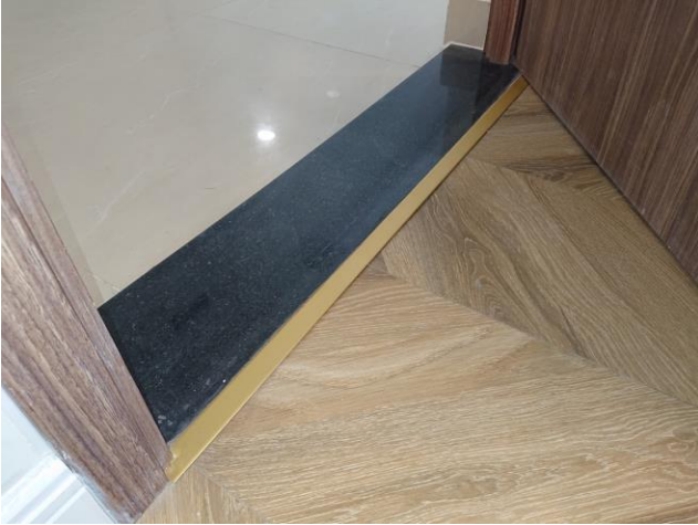
■ CONDOMINIUM (HO CHI MINH/VIETNAM)
