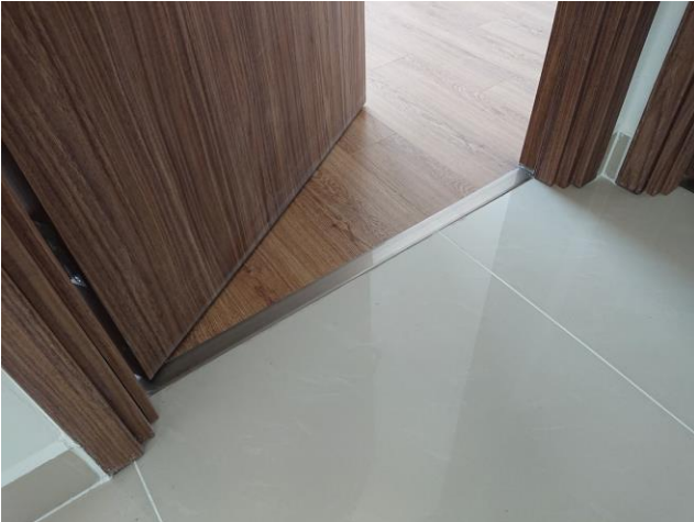
■ CONDOMINIUM (HO CHI MINH/VIETNAM)
